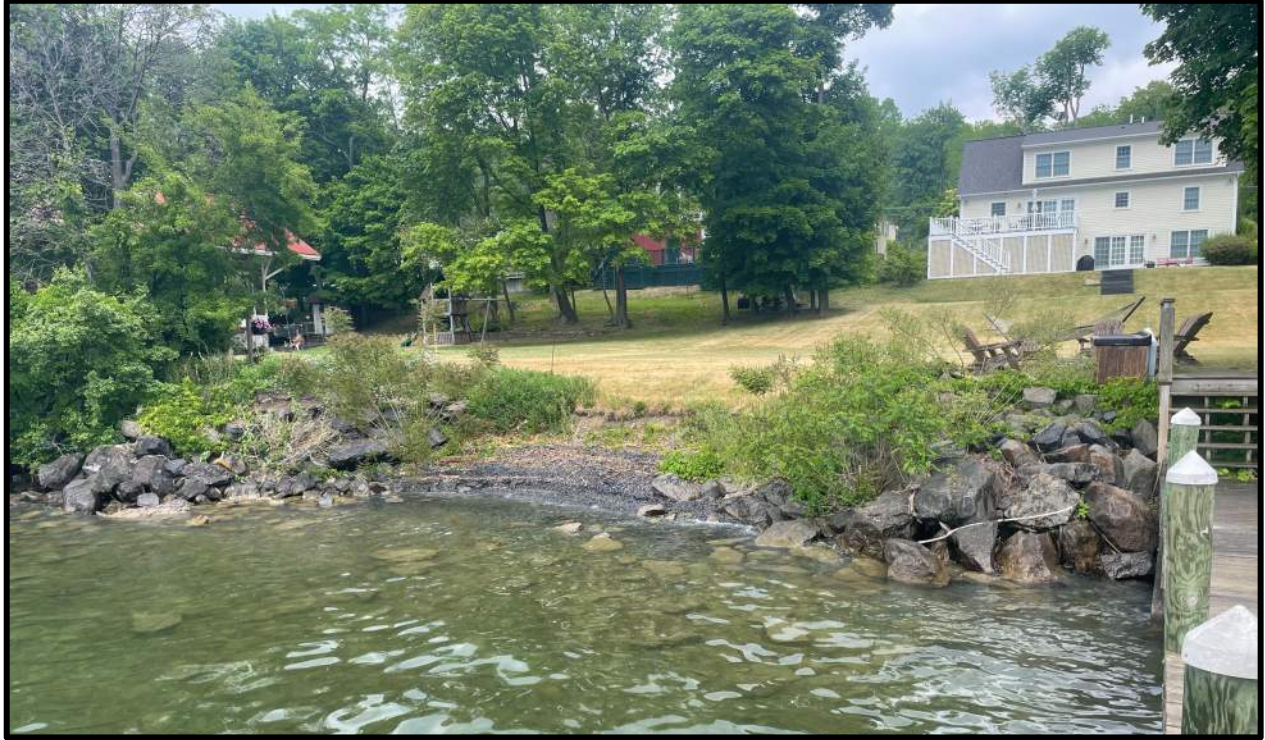
Photo of Existing Shoreline North of Dock
