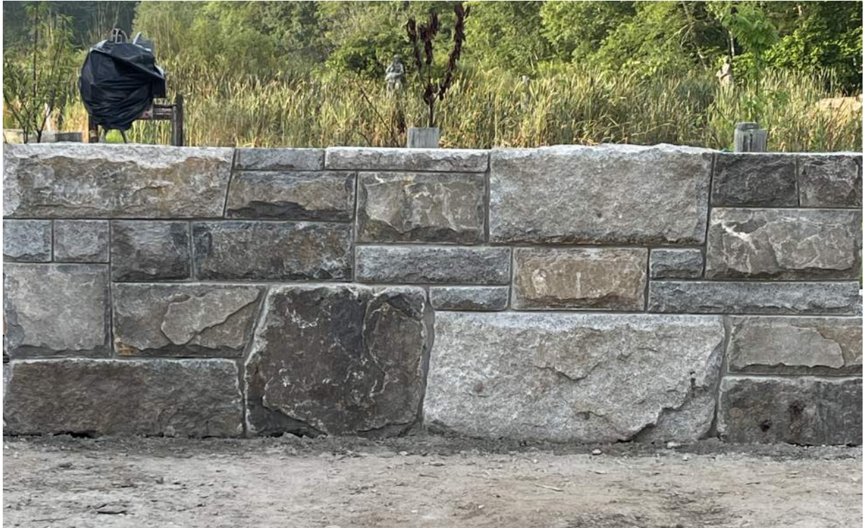
Mockup of Proposed Wall With Deep Raked Joints
